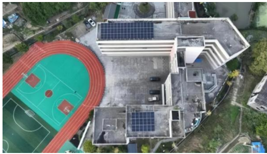
Figure: CZBank cooperated with CHINT Energy's "One kWh Electricity" Public Welfare Foundation to donate campus photovoltaic power stations
