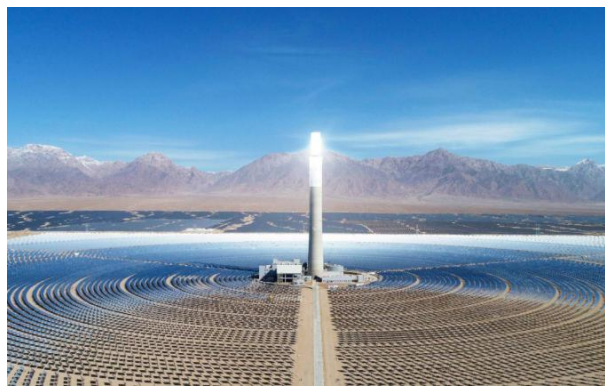
Figure: Overview of tower molten salt energy storage and solar thermal project constructed by Cosin Solar
